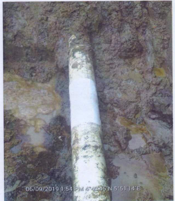
FIG D: Incident point after repairs
