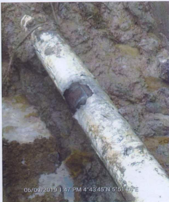
FIG C: Incident point after repairs (patch plating)
